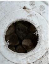
\*Fill bucket with river rock through the hole in the top of the bucket. (Leaving some room at the top will help it from overflowing when gray water is dumped. Step 4:
