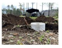
\*Rake dirt and rock around bucket and the goal is to have 1" to 2" of the bucket visible.
